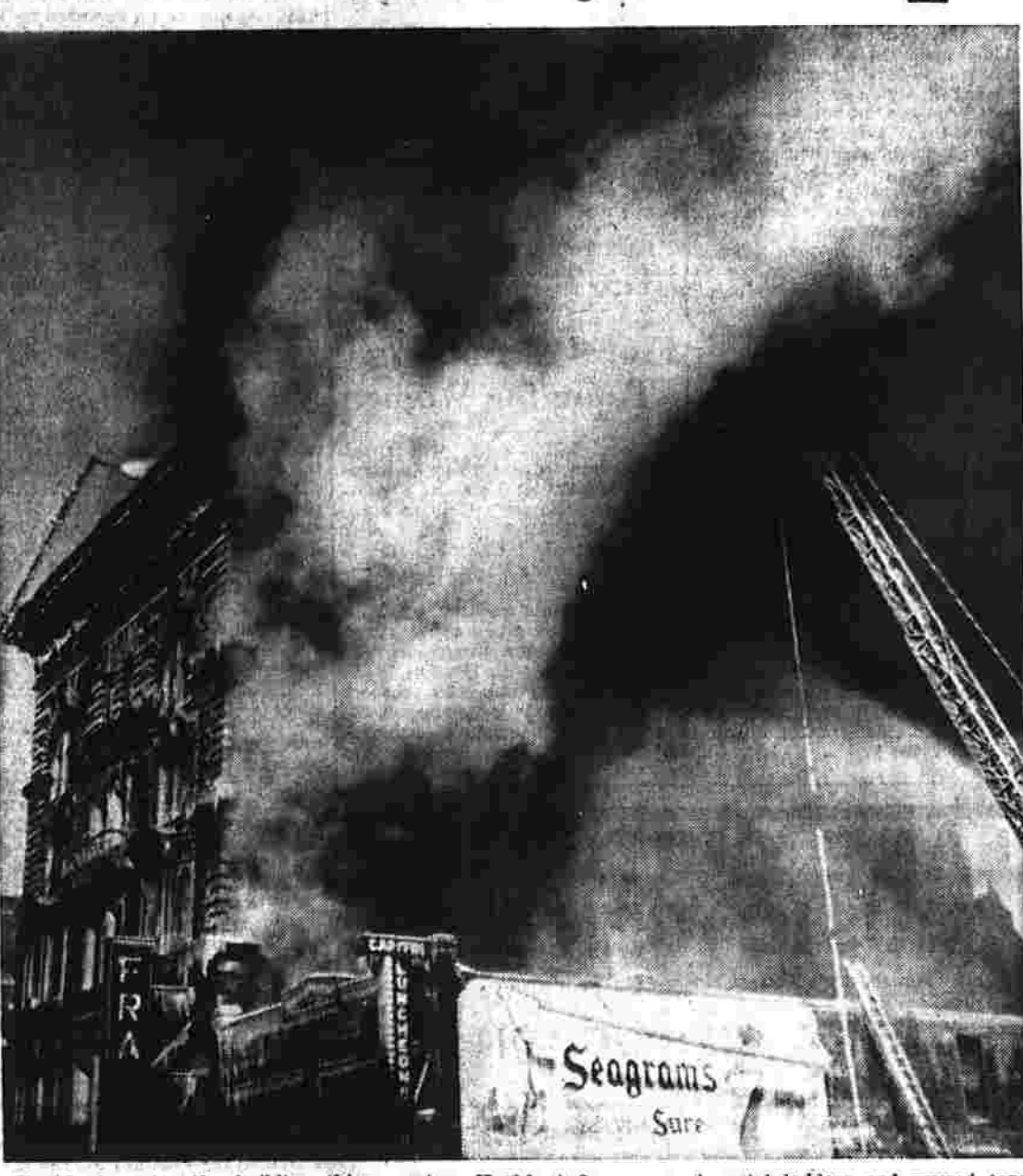
Unable to enter the building this morning, Hartford firemen used aerial ladders and poured tons of water on this six-story structure at Asylum and Ann Sts. It appeared that loss might reach $500,000. (Herald photo by O'Neil).
